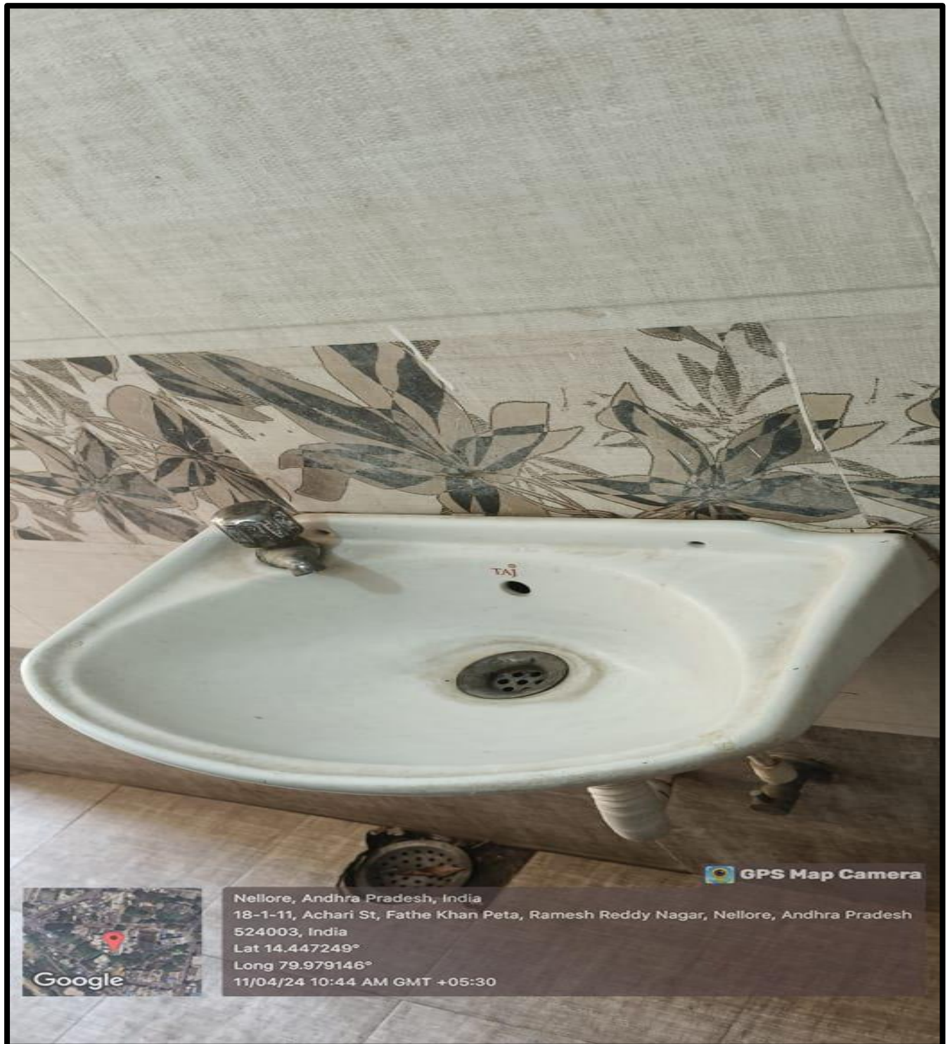
Figure : Usage of Waste water for hand wash
